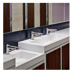
With the Dyson Airblade Tap hand dryer, hands can be both washed and dried at the sink. There's no need to move to a separate drying area, so water isn't dripped on the floor.
